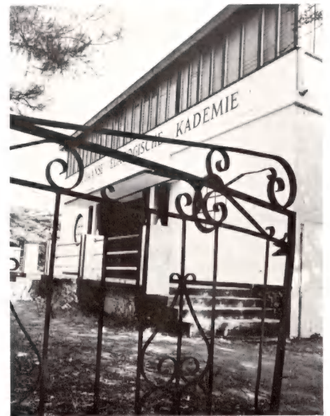
The Mansur Building
